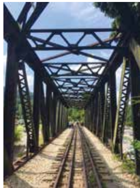
Bukit Timah Railway Bridge
